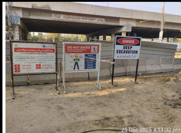
Hard Barrication & Signages
