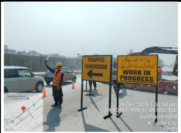
Flagman & signages during trail pits
