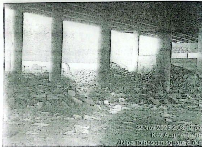
Figure 2 Excavated Earth stacked under the SSUET Flyover
