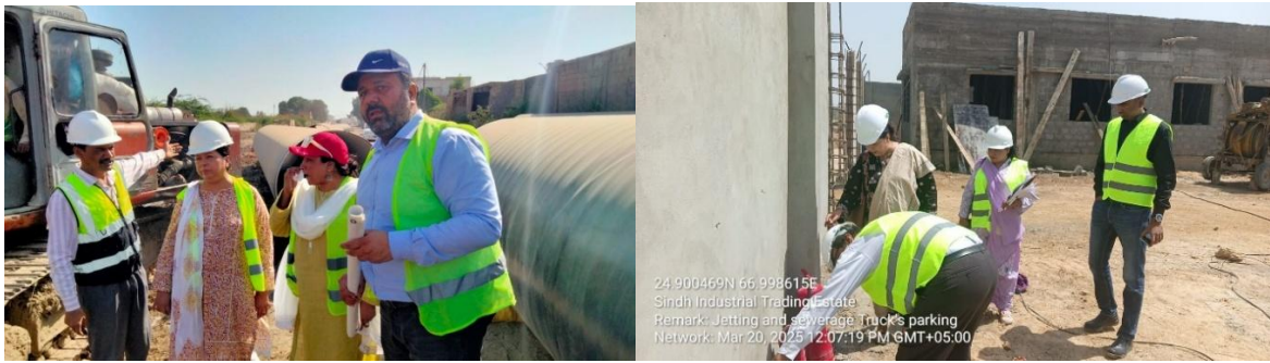
Field visit parking sheds
