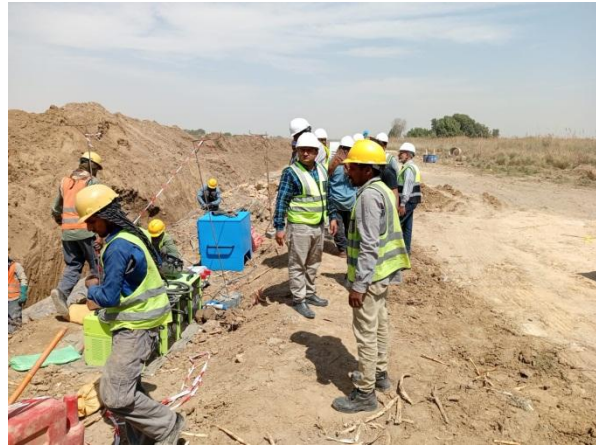
The workers were seen with required PPE's
