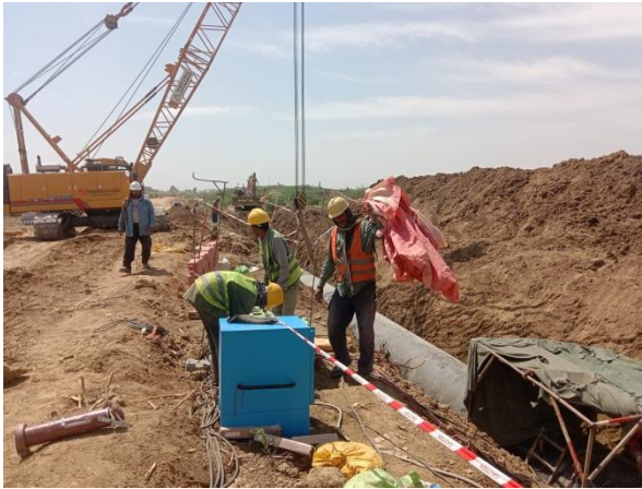
The excavated trench was seen with tap barricading measures
